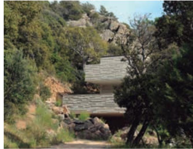
In France, for example, we added tuff, a dust from some Bonifacio stone, to a mixture of cement, sand and stone, so that the resulting colour of the concrete would blend in with the surrounding nature. We also poured this concrete into moulds fitted with wooden planks of different thicknesses. This resulted in a grooved effect and also created flat horizontal parts where vegetation debris and marine sediments could be deposited.
