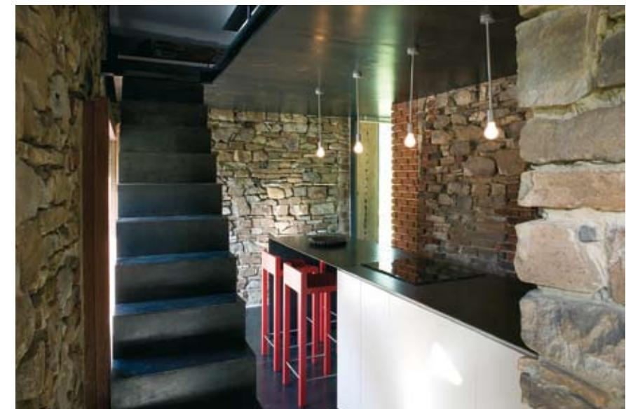
Apart from the steel sheets on the ground, other such sheets are folded to create the kitchen work top, the stairs and the flooring on the first floor.
